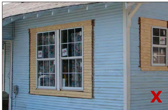
Do not reduce historic window openings to fit stock window sizes or use faux divided lights when replacement is necessary. (Photo: Ron Bauml, San Antonio Conservation Society)
