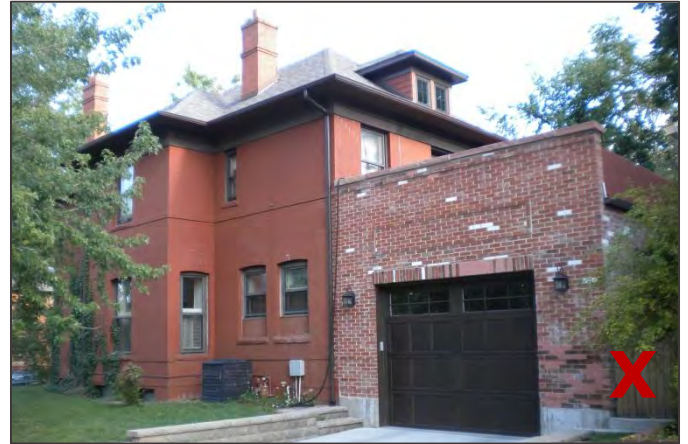
This new garage is not consistent with the material or character of the historic home.
