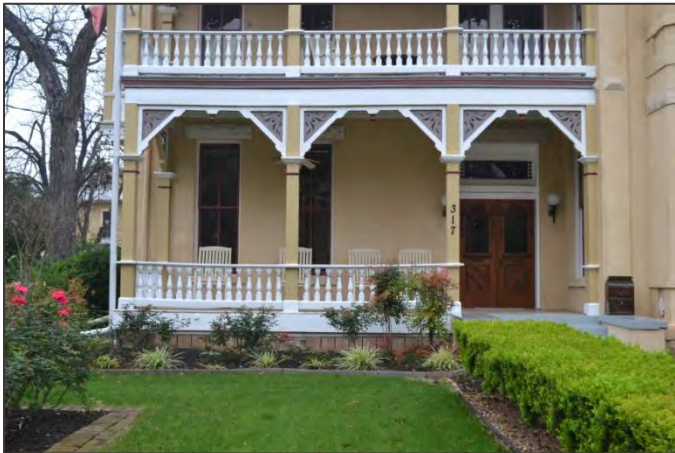
The architectural detailing of this porch has been preserved.
