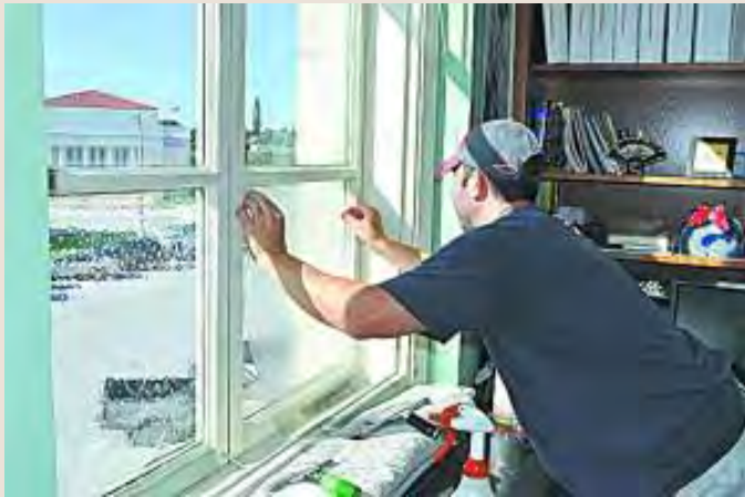
Applying solar window film can block more than half of the solar heat that would otherwise enter the building. (Photo: Belkys Perez, Coral Gables Community Newspaper)
