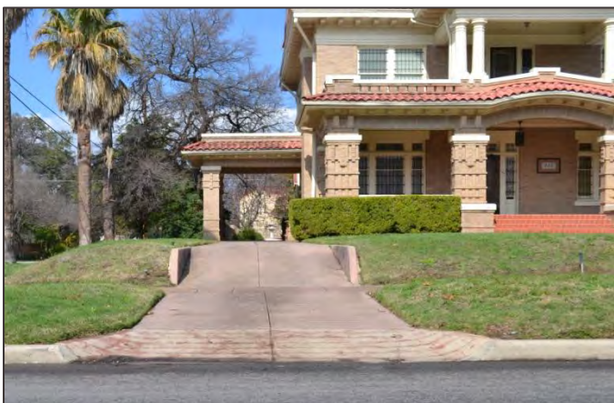
This historic porte-cochere matches the primary structure in form, detailing, and materials.
