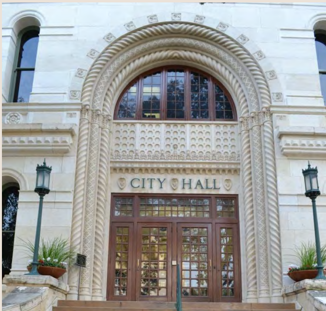
The fanlight, detailing, and glazed area of this entrance help define the character of this public building.
