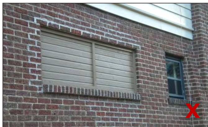
Do not alter the character and symmetry of the façade by filling historic window openings.
