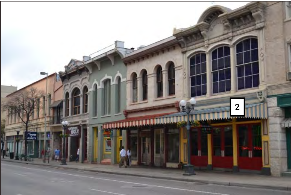
Typical canopies and awnings in San Antonio's historic districts include both metal storefront canopies and fabric awnings.
