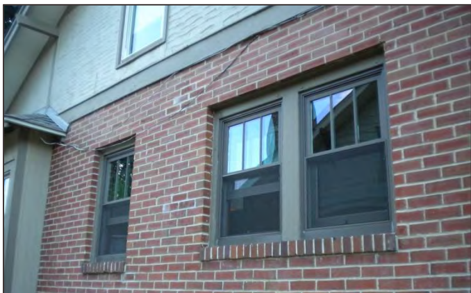
Use the exterior muntin pattern, profile, and size appropriate for the historic building when replacement windows are necessary.
