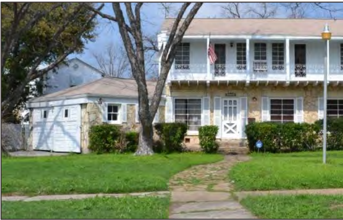
These highly visible garage doors were replaced with doors similar in character to the ones beyond repair.
