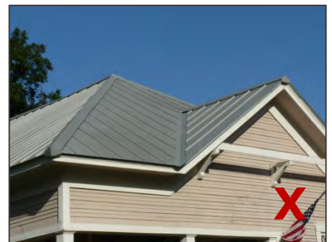
Do not use ridge caps with ridge cap vent (left) or end caps (right).
