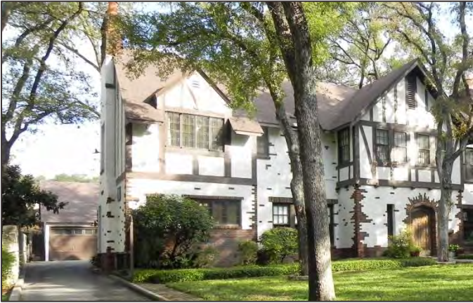
This new garage is discretely located behind the primary structure and is designed to match its historic character.
