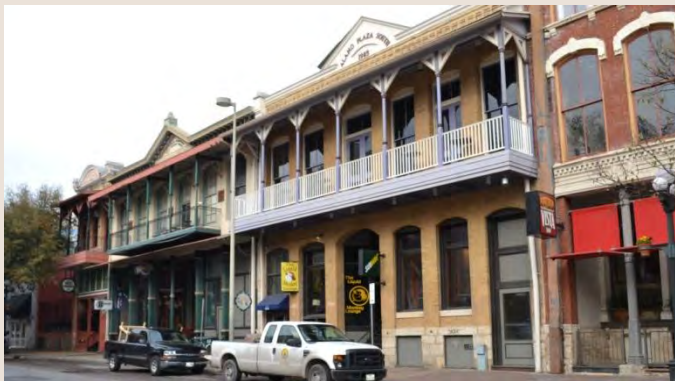
These downtown buildings feature full-width cantilevered balconies with decorative woodwork.
