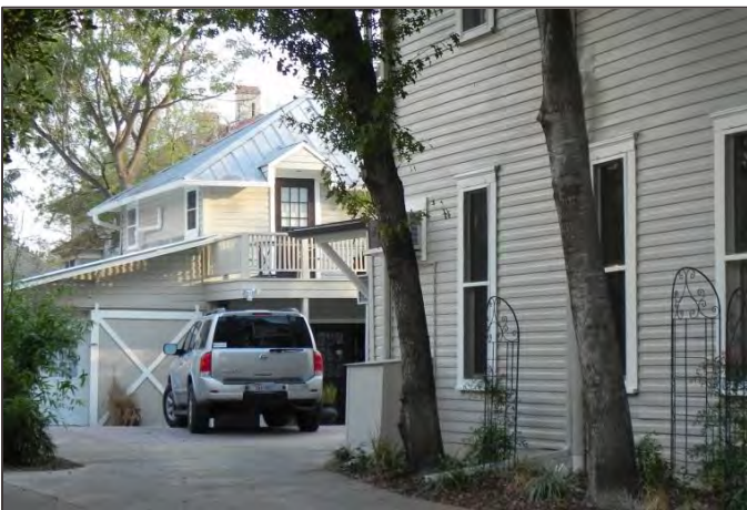
This historic garage has been sensitively modified to incorporate a modest accessory dwelling above it.
