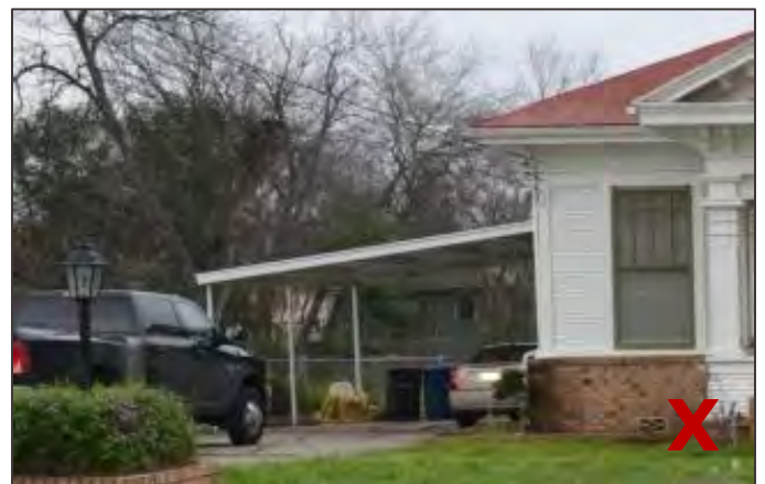
This carport has been added to this historic building to serve the same function as a historic porte-cochere, but distracts from the building's character.
