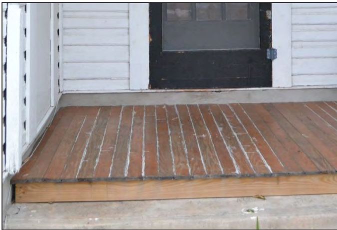
Original wood flooring on this porch is in good condition and will continue to be with proper maintenance.
