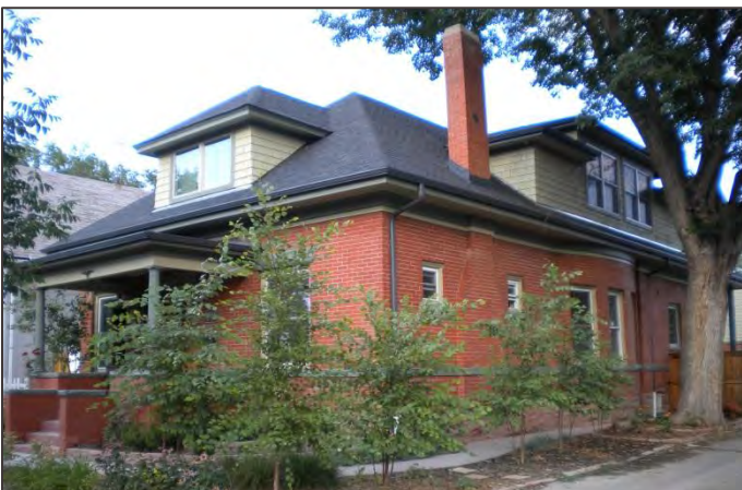
A side dormer addition with similar roof forms and architectural details complements, but doesn't detract from, the character of the original structure.
