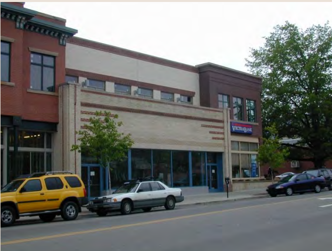
The upper-story addition (center) in this neighborhood commercial district incorporates complementary, yet varied, materials to protect the character of the surrounding historic district.
