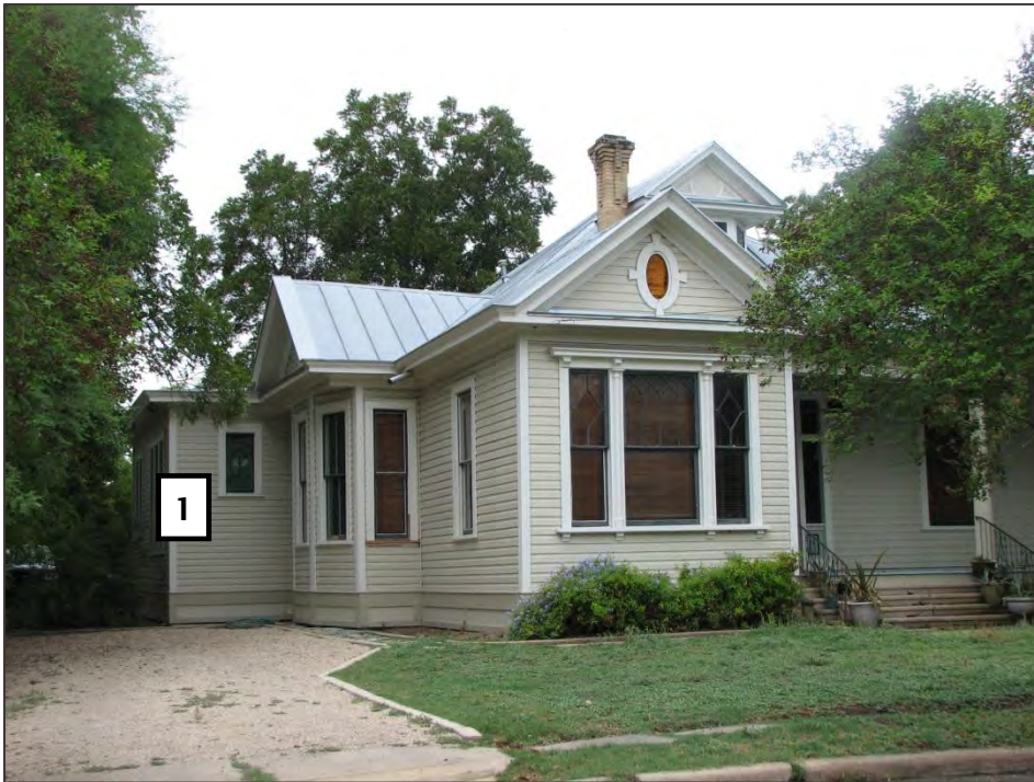
This rear addition complements architectural details found on the primary historic structure.
