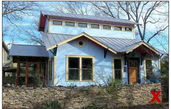
The scale and placement of this inappropriate second story addition overwhelms and obscures the form and character of the original structure.
