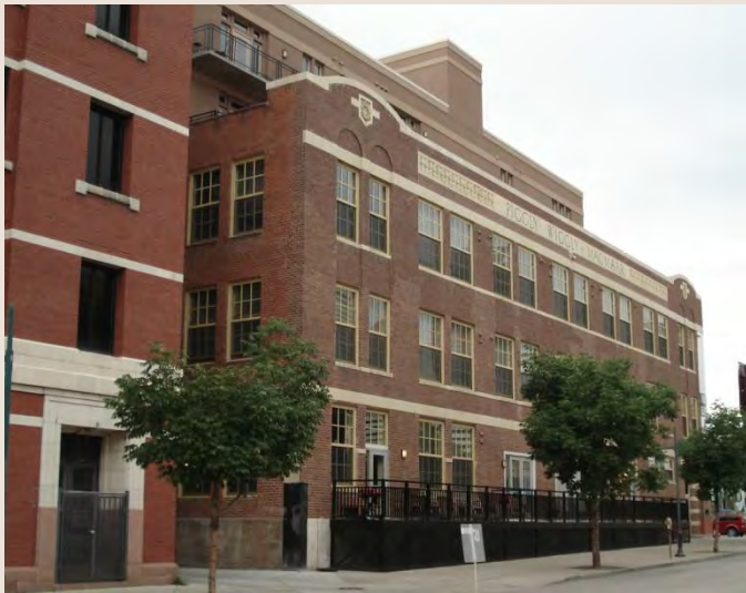
A fourth floor addition to this historic building is set back from the primary façade, minimizing its visibility from the public right-of-way.
