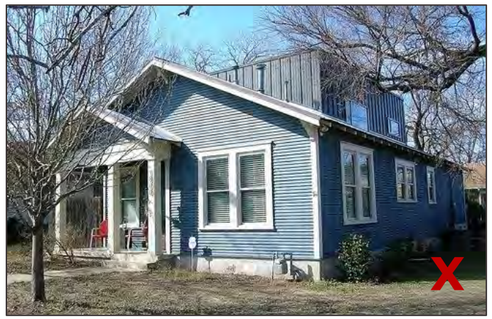
This dormer addition varies dramatically in form and materials from the original structure and is clearly visible from the public right-of-way.
