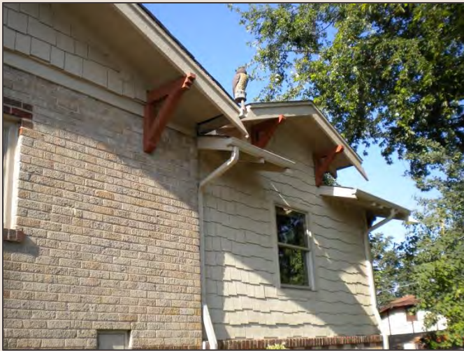
The use of contrasting, but complementary, materials and a modest offset for this rear addition provides a clear transition between old and new building elements.
