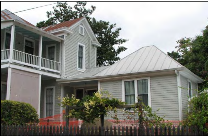
This addition is sited below the peak of the roof and is scaled so as not to alter the appearance of the home's front façade or otherwise detract from the original structure.
