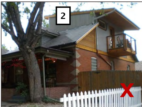
These additions detract from, rather than complement, the character of the primary historic structures due to the use of incompatible roof forms, massing, and architectural details.
