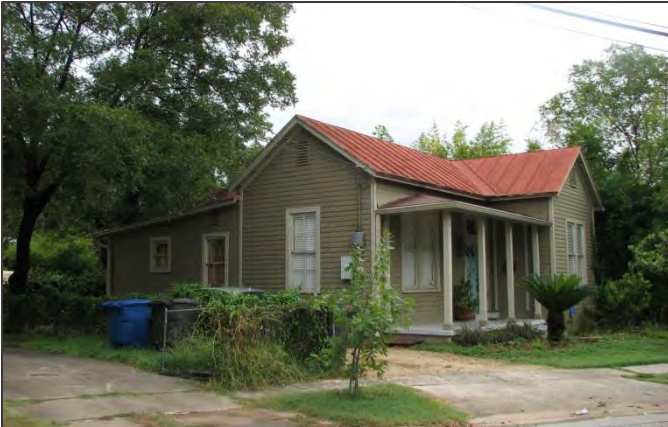
A modest setback combined with compatible, but varied, roof forms distinguishes this rear addition (left) as new without distracting from the character of the original structure.
