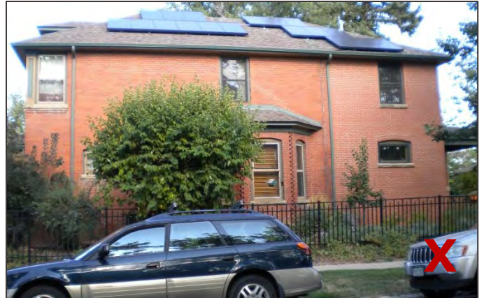
A lack of variation in roof form, height, and massing blurs the line between this rear addition (right) and the original structure.
