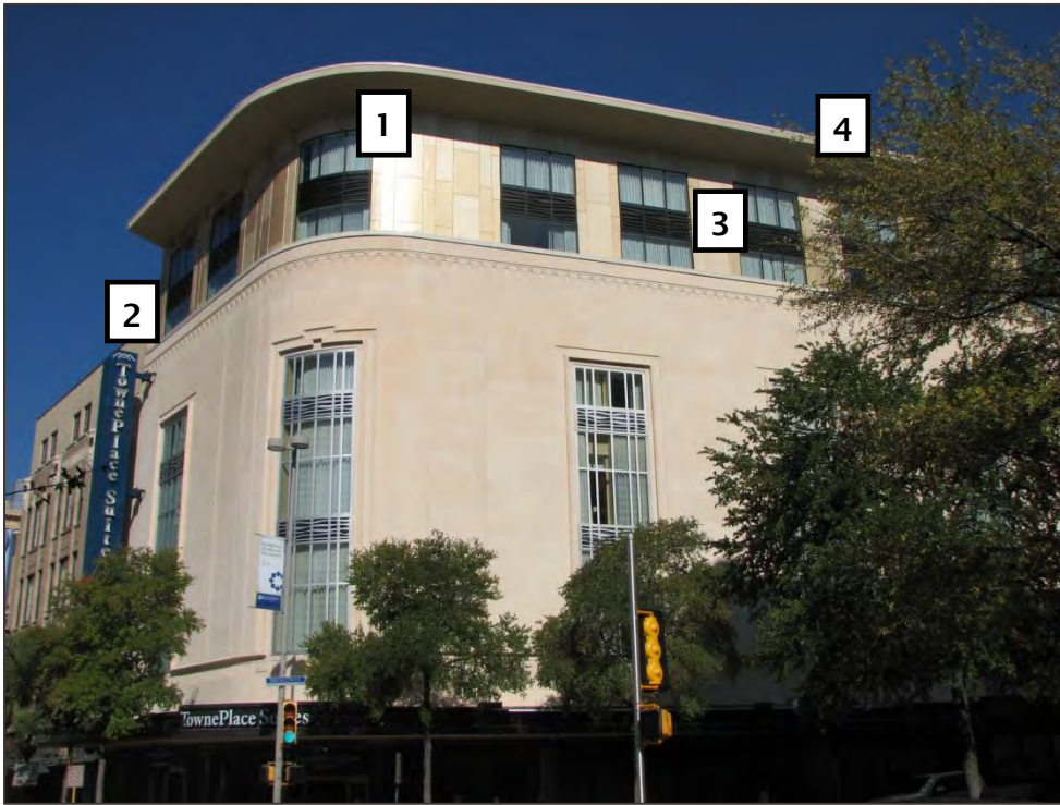
A second story addition to this commercial storefront is set back from the primary façade and is distinguishable from the historic building.
