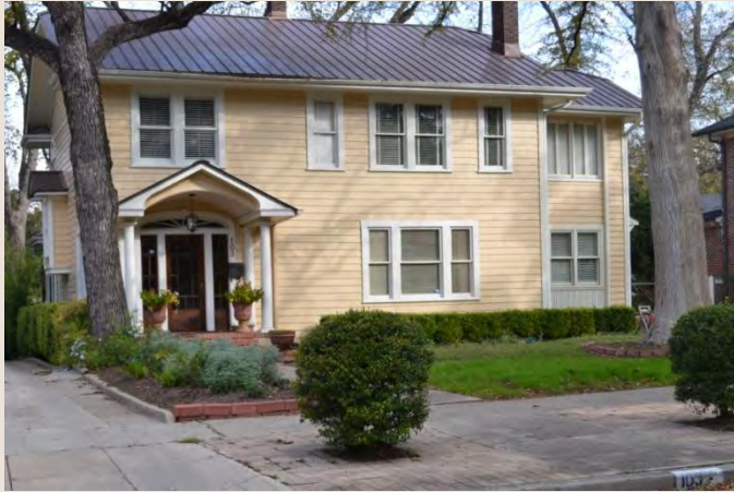
An addition to this residence (visible at far right) is setback from the primary façade, clearly distinguishing it from the primary historic structure.
