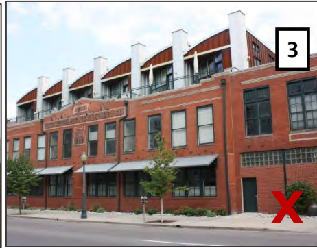
These additions detract from, rather than complement, the character of the primary historic structures due to the use of incompatible roof forms, massing, and architectural details.
