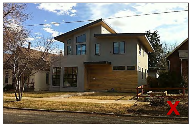
A side-oriented entrance and blank street level façade on this new home conflicts with the pattern established by historic homes along the street frontage.
