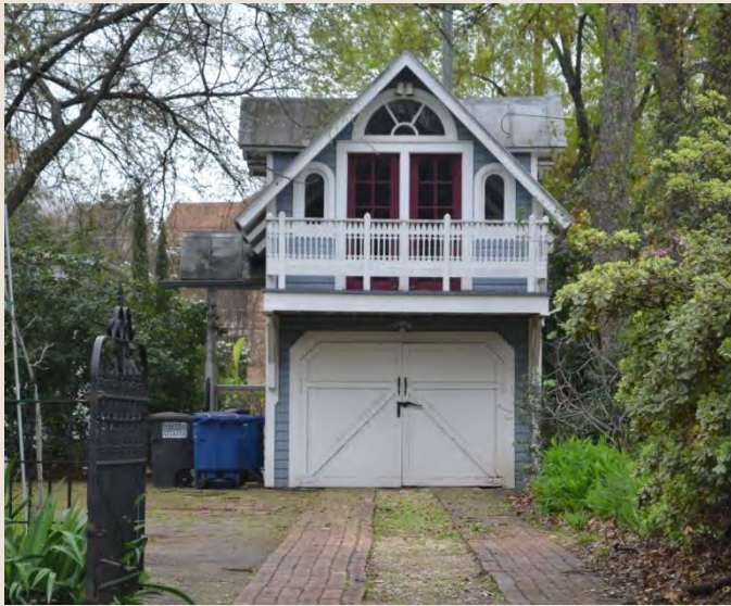
The architectural features of this outbuilding are similar in character to the primary historic building.
