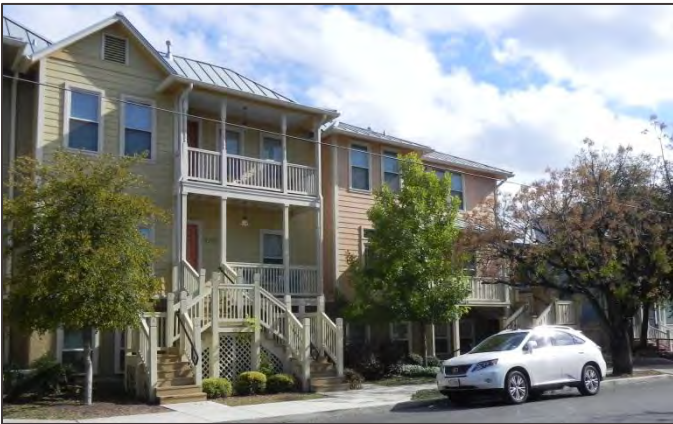
Entrances and front porches on this new multi-family project are oriented towards the street, consistent with nearby historic homes.
