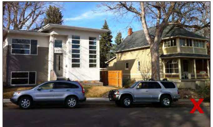
Although the scale and massing of the new home (left) is compatible with historic homes on the block, the ratio and placement of windows to walls and foundation and floor heights varies considerably.
