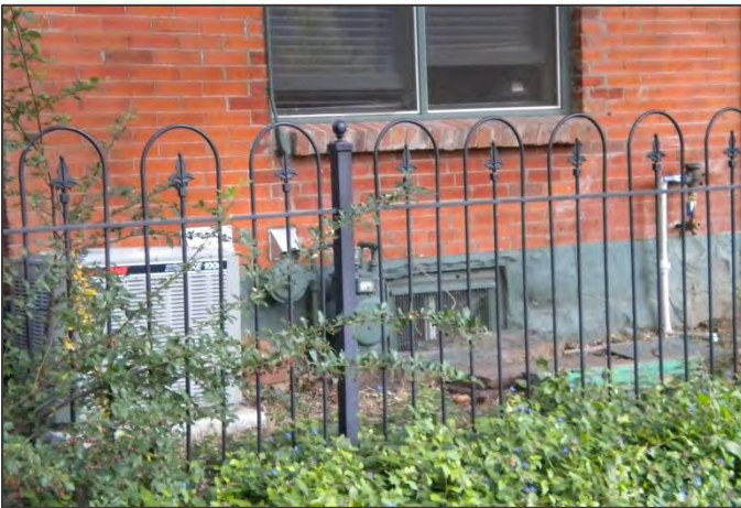
Air conditioning units should be located in a rear yard or along a secondary façade and screened from view.
