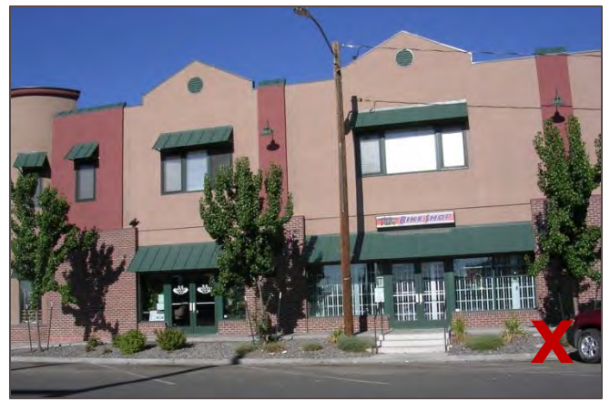
This new structure lacks sufficient architectural detail to be appropriate within a historic district.
