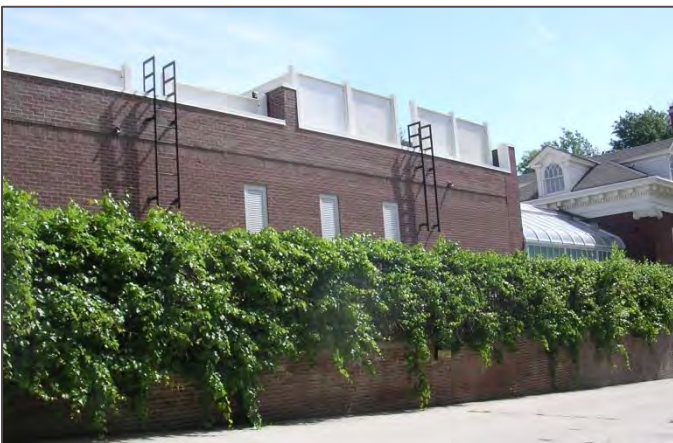
Rooftop mechanical equipment on this addition to a historic structure is screened from the public right-of-way.
