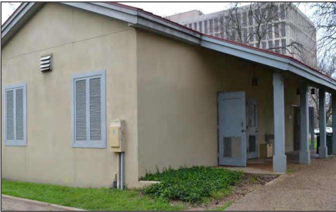
This utility box is located on a secondary façade and painted to match the color of the primary historic structure.
