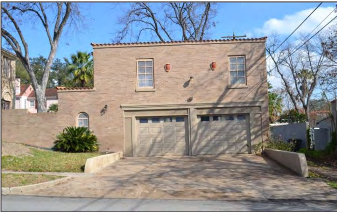
This new garage and accessory dwelling unit have been designed using compatible materials and architectural details to complement the primary structure.
