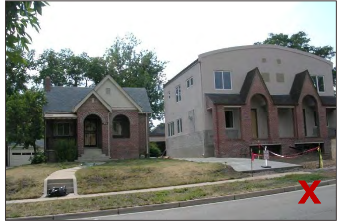
The new structure (right) unsuccessfully attempts to achieve compatibility by mimicking historic design elements found on surrounding homes in the district while disregarding issues of scale and massing.
