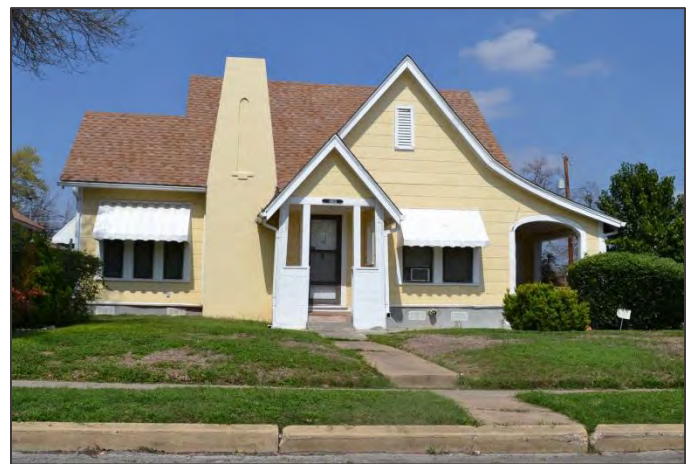
Tudor Revival Style bungalow, Keystone Park Historic District.
