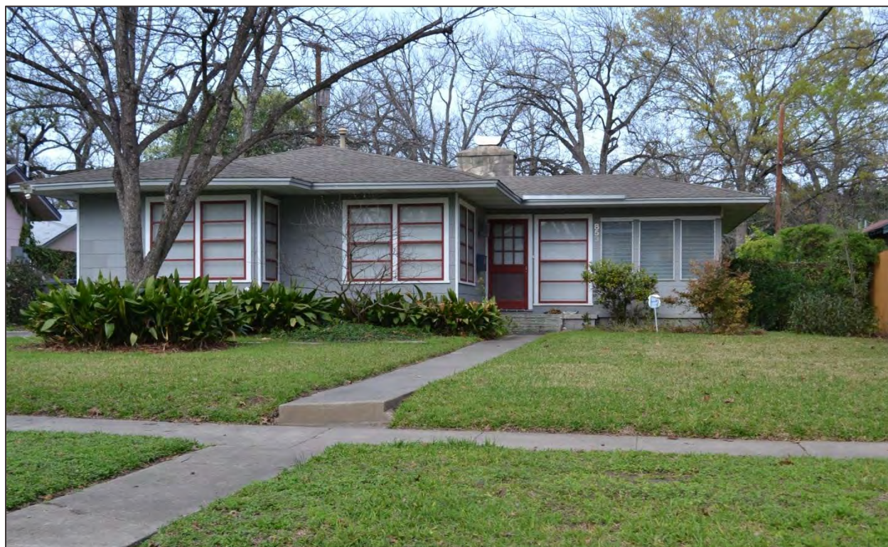
Ranch house, River Road Historic District. Note the low slope of the roof, the deep overhanging eaves, the wood-sash awning windows at the right, and the metal-sash jalousie windows at the left.
