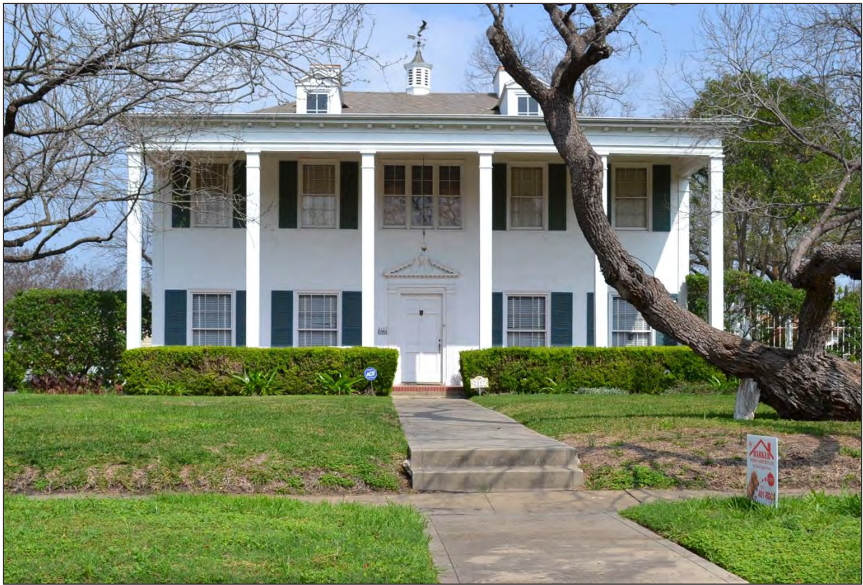
Colonial Revival house, Monticello Park Historic District. Note the pediment over the door.
