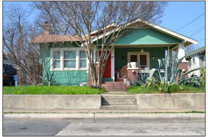
Concrete retaining wall, Tobin Hill Historic District. Note the sidewalk immediately adjacent to the street.
