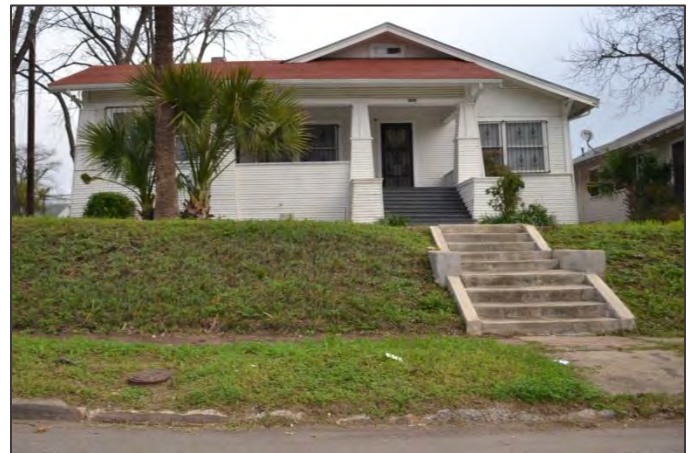
Craftsman Bungalow, Knob Hill Historic District. Note the slope of the lawn and the walkway.
