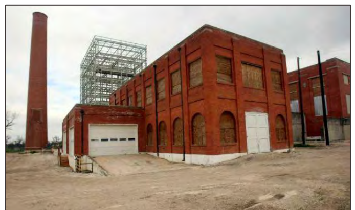
Mission Road Power Plant, Mission Historic District. Source: www.mysanantonio.com .
