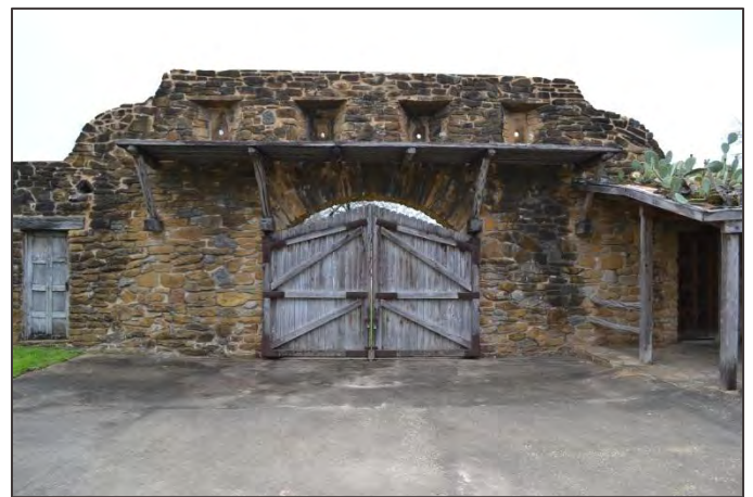
Perimeter wall and gate, Mission San Juan, Mission Historic District.
