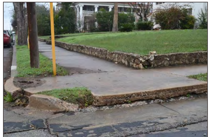
Historic concrete curbing and stone retaining wall at W. French Place and Belknap Avenue.
