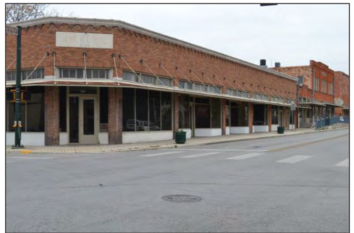
Commercial buildings along New Braunfels Avenue, Government Hill Historic District.
