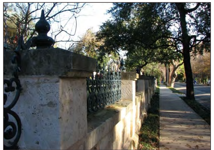
Stone wall with wrought iron detail, King William Historic District.
