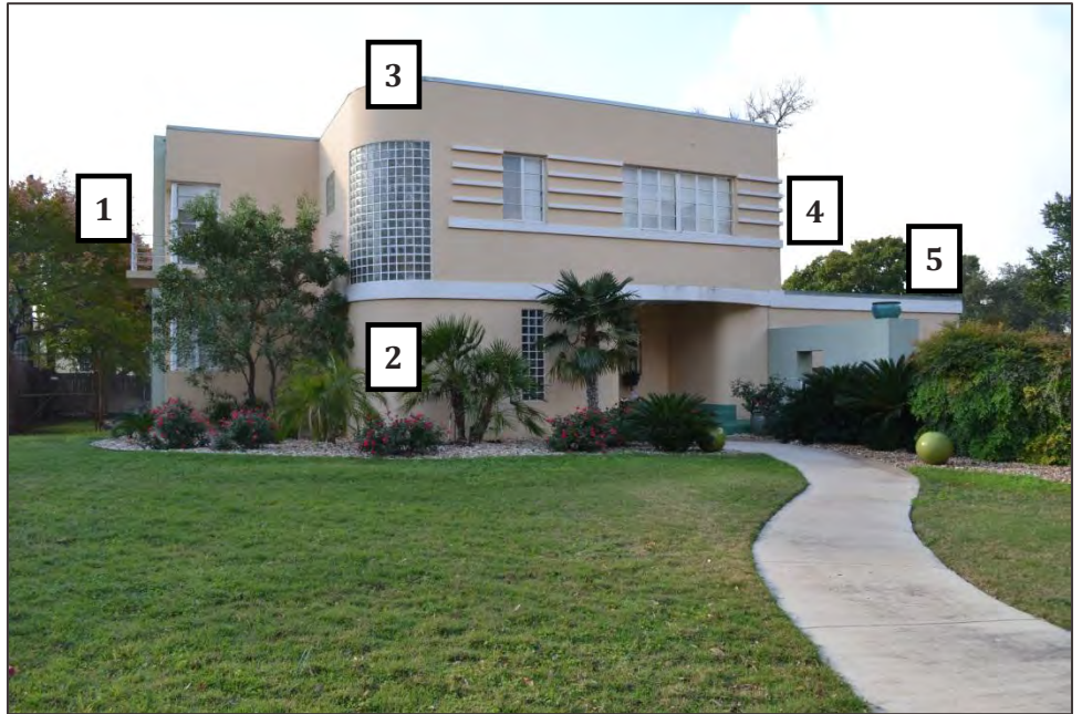
Moderne house, Monte Vista Historic District.
