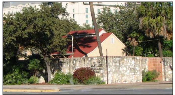
Perimeter wall, S. Alamo St. at E. Nueva Street, La Villita Historic District.
