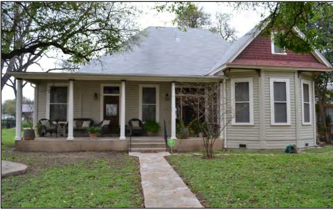
Folk Victorian house, Mission Historic District. Note that the original porch floor and stoop likely were wood.
