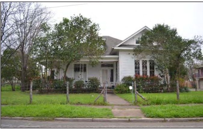
Folk Victorian house, Lavaca Historic District. Note that the original porch posts likely were wood.
