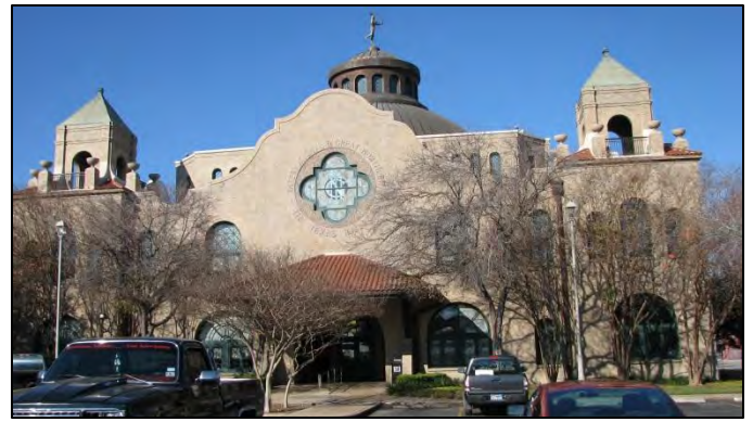
View of the former I&GN Railroad Depot, Cattleman Square Historic District.
