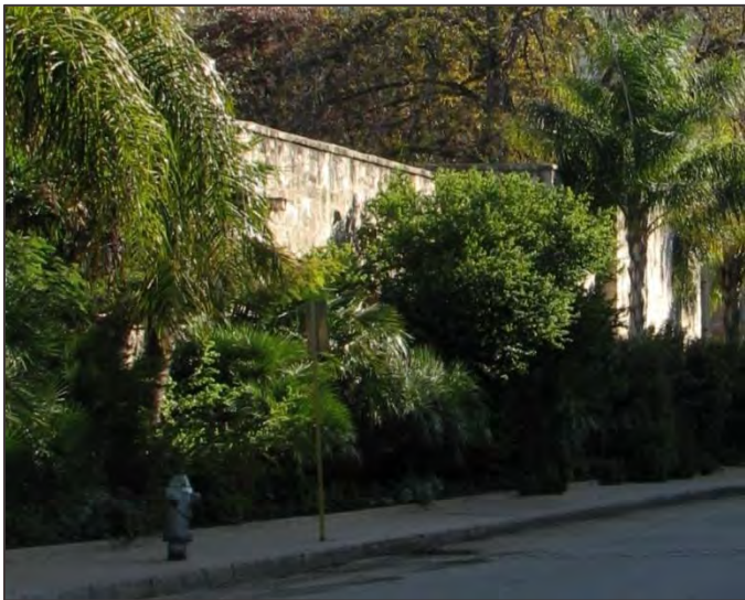
Detail of the stone wall along the southern perimeter of the Alamo.
