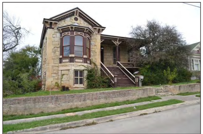
Brick retaining wall, 500 block of Burleson Street.
