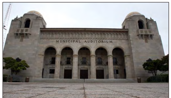
Municipal Auditorium, Auditorium Circle Historic District. Note the front plaza and the Spanish Colonial Revival detailing. Source: blog.mysanantonio.com .
