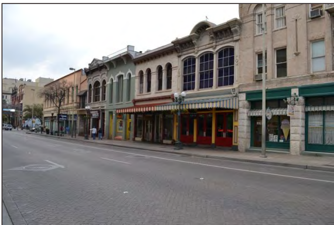
Streetscape in the Alamo Plaza historic district along E. Commerce St. illustrating buildings set forward flush to the lot line and sharing party walls with the neighboring buildings.
