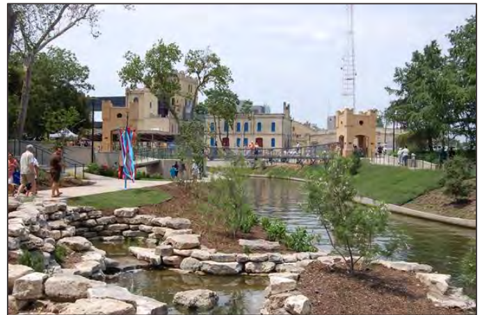
View of the Old Lonestar Brewery from the Museum Reach of the San Antonio River Walk. Source: http://www.sanantonioriverwalk.com/museumreach.html .
