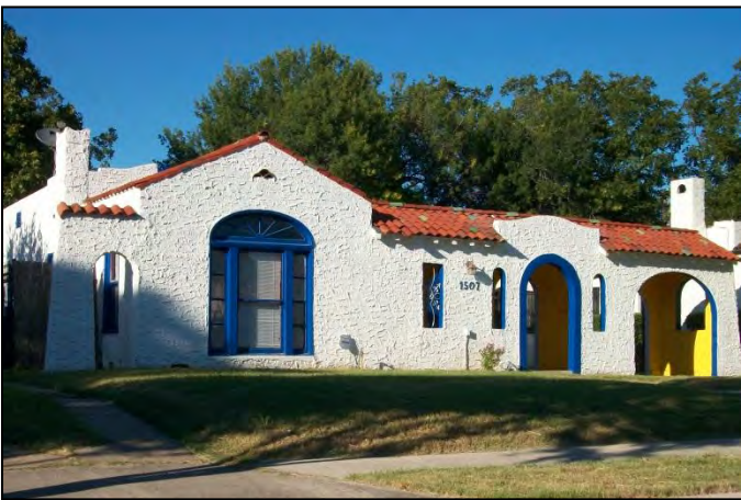
Spanish Eclectic house, Fulton Avenue Historic District.
