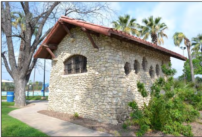
Restroom building, Woodlawn Lake Historic District.
