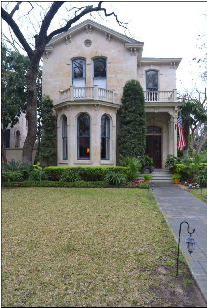
Italianate House, King William Historic District. Note the segmental-arched window lintels and bay window with a flat roof.
