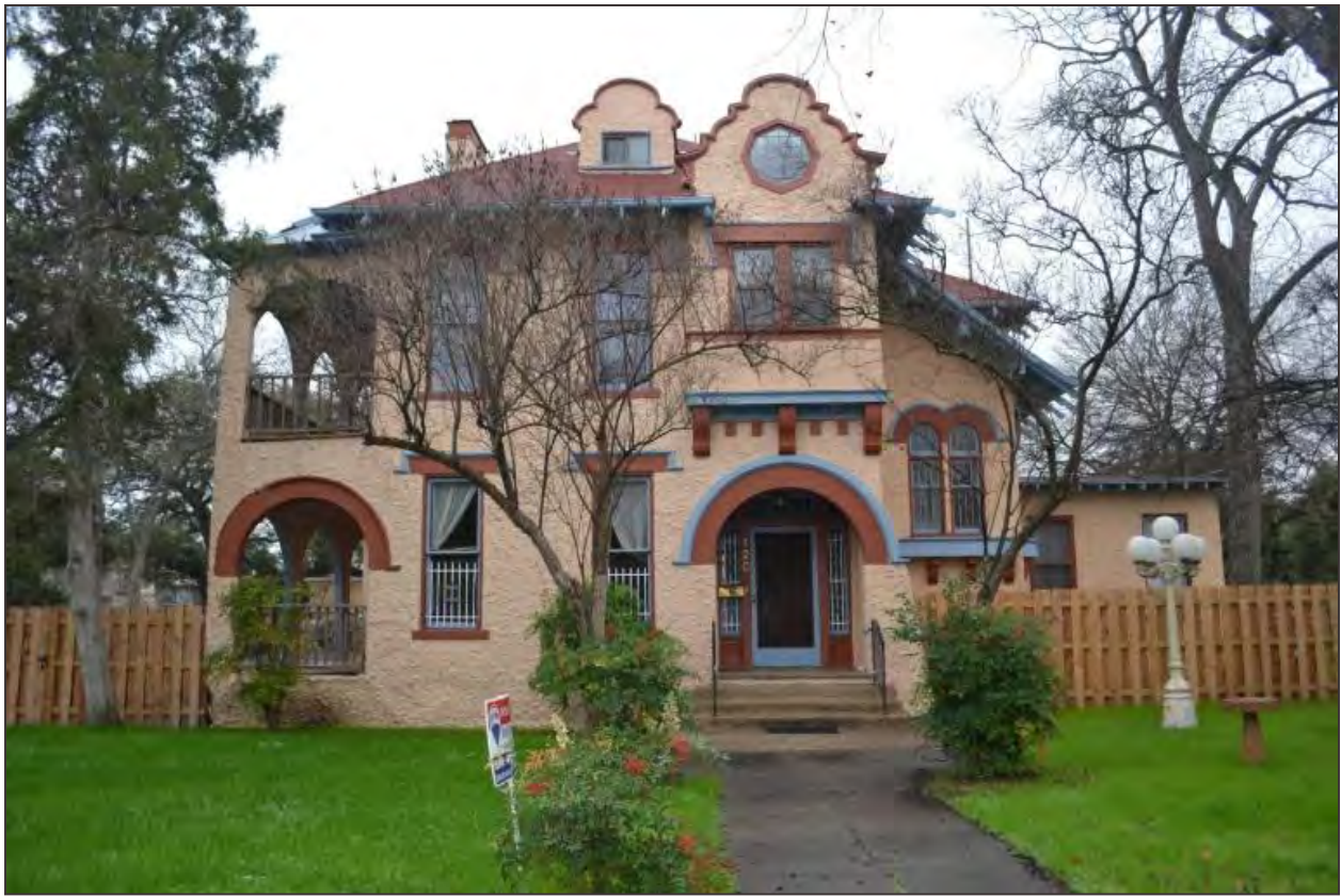
Mission Revival Style house with molded parapet, round-arched entry and doors, and loggia at side porch, Monte Vista Historic District.
