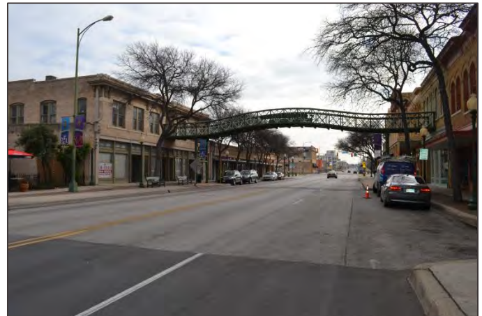
Streetscape view, E. Commerce Street, St. Paul Square Historic District. Note the archway, setbacks, and lighting.
