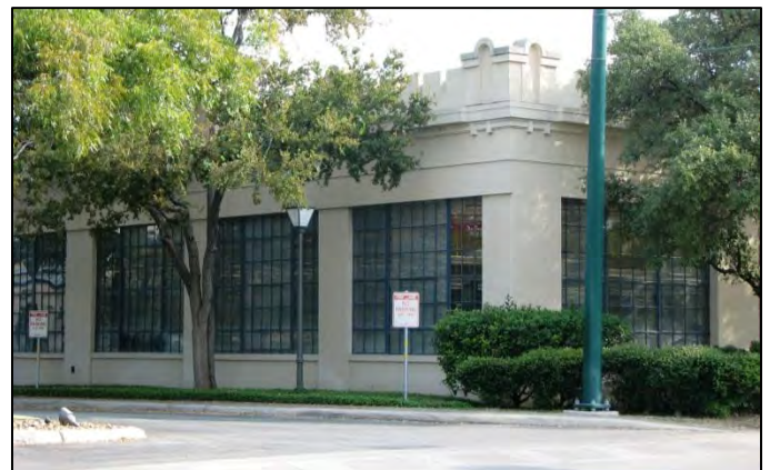
View of the Arsenal at the main entrance drive.
