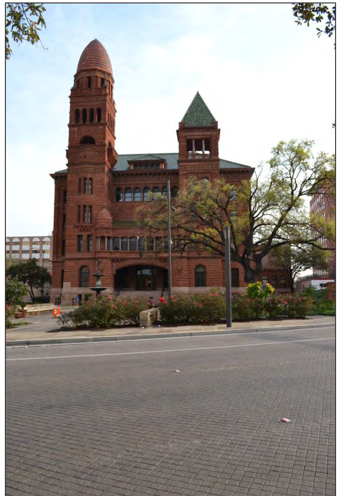
Romanesque Revival Style Bexar County Courthouse, Main and Military Plaza Historic District.
