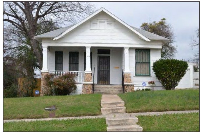
Craftsman bungalow with tapered stone piers at porch, Dignowity Hill Historic District.
