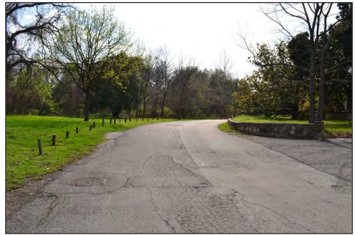
View looking south along River Road, River Road Historic District.
