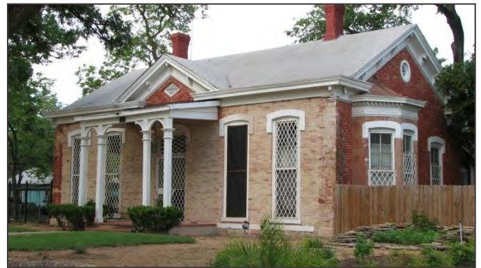
Dignowity Hill residence, N. Olive Street.
