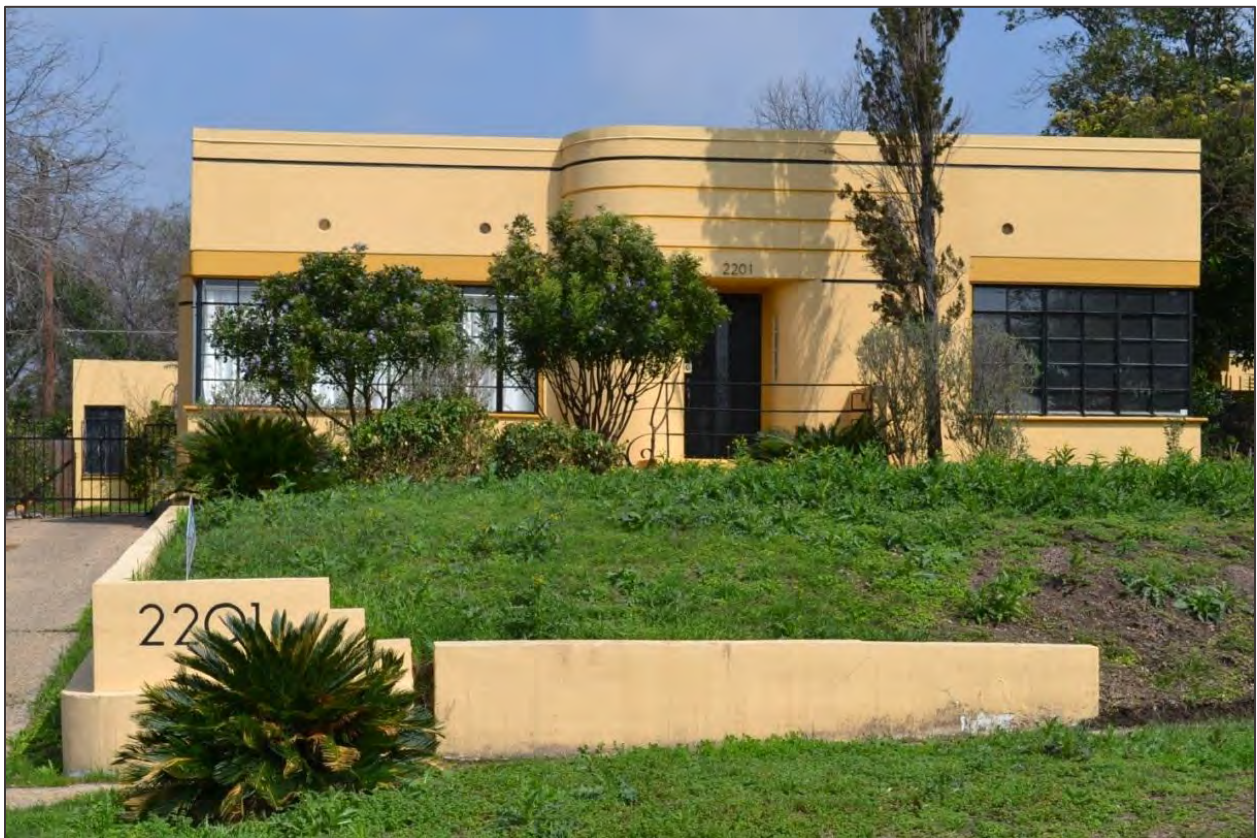
Moderne house, Monticello Park Historic District.
